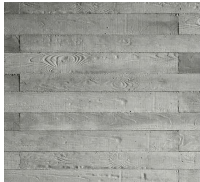
CT-01 Board-Formed Concrete
